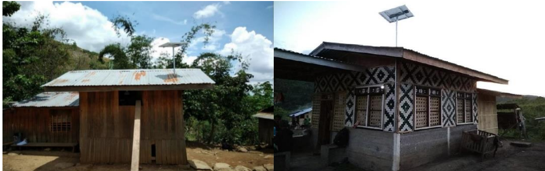
Diagram 7 : Roof-through Pole mounted installations on GI roofs
